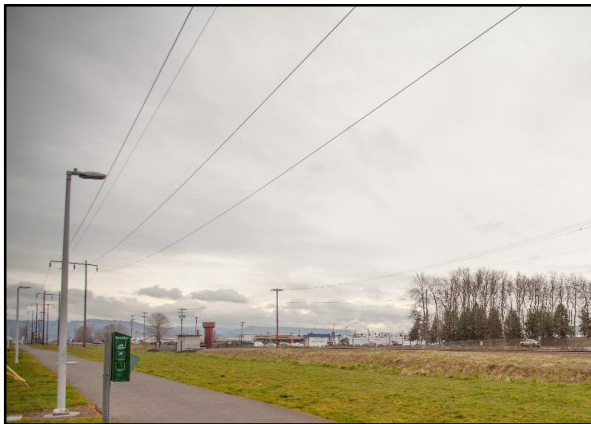
Photo 5: BPA transmission lines along CDID Ditch No. 3.
